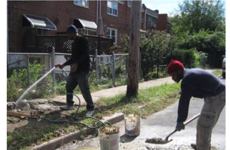
LACK OF TRUST TOWARDS PUBLIC WORKS Residents taking into their own hands to do sidewalk repair; the sidewalk was heaved up by the roots of a sheet tree.
